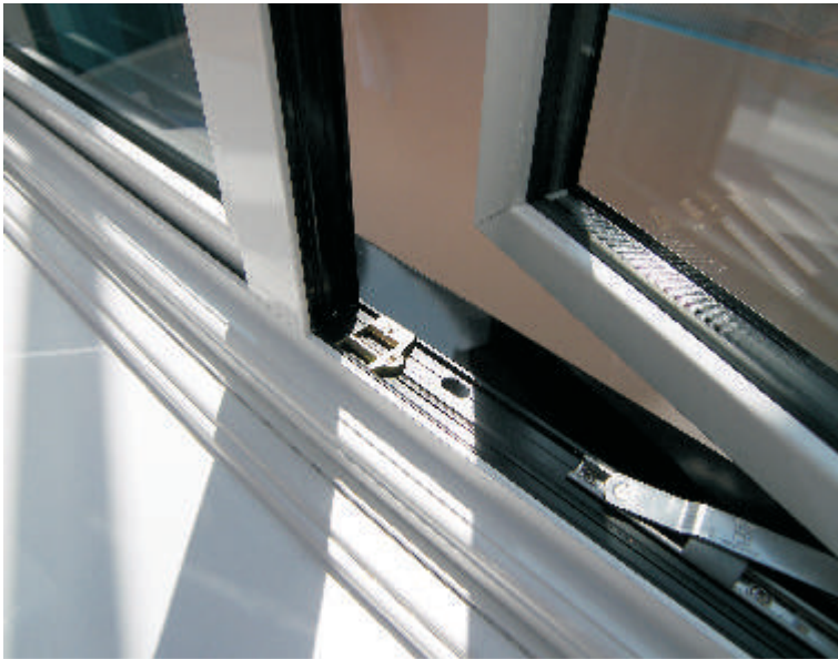
Above picture shows dummy vent next to opener, black outside and white inside.
